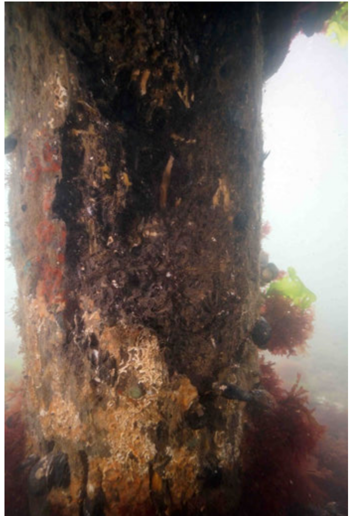
Pile 24D: Poor Condition – 50% loss of section within tidal zone
