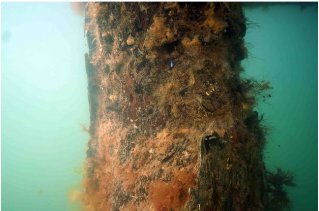
Pile 44C: Poor Condition – 40% loss of section – lower tidal zone. Top-end splitting
