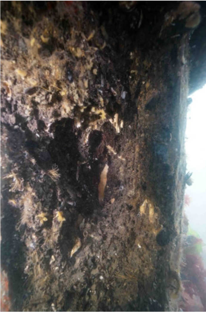
Pile 25C: Poor Condition – 40% loss of section within tidal zone. Severe hallowing
