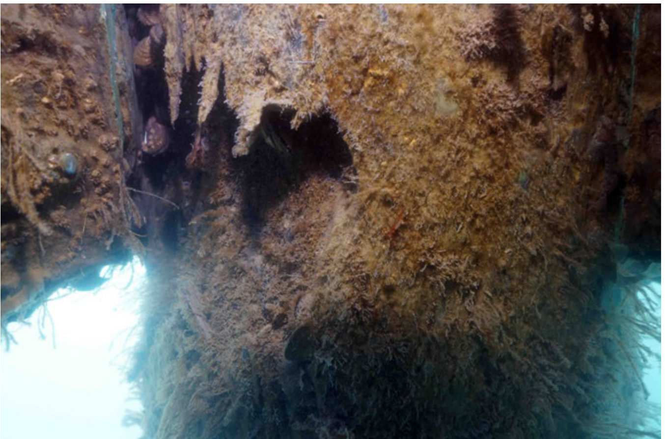
Pile 38D: Poor Condition – 35% loss of section – above tidal zone. Moderate hollowing & decay
