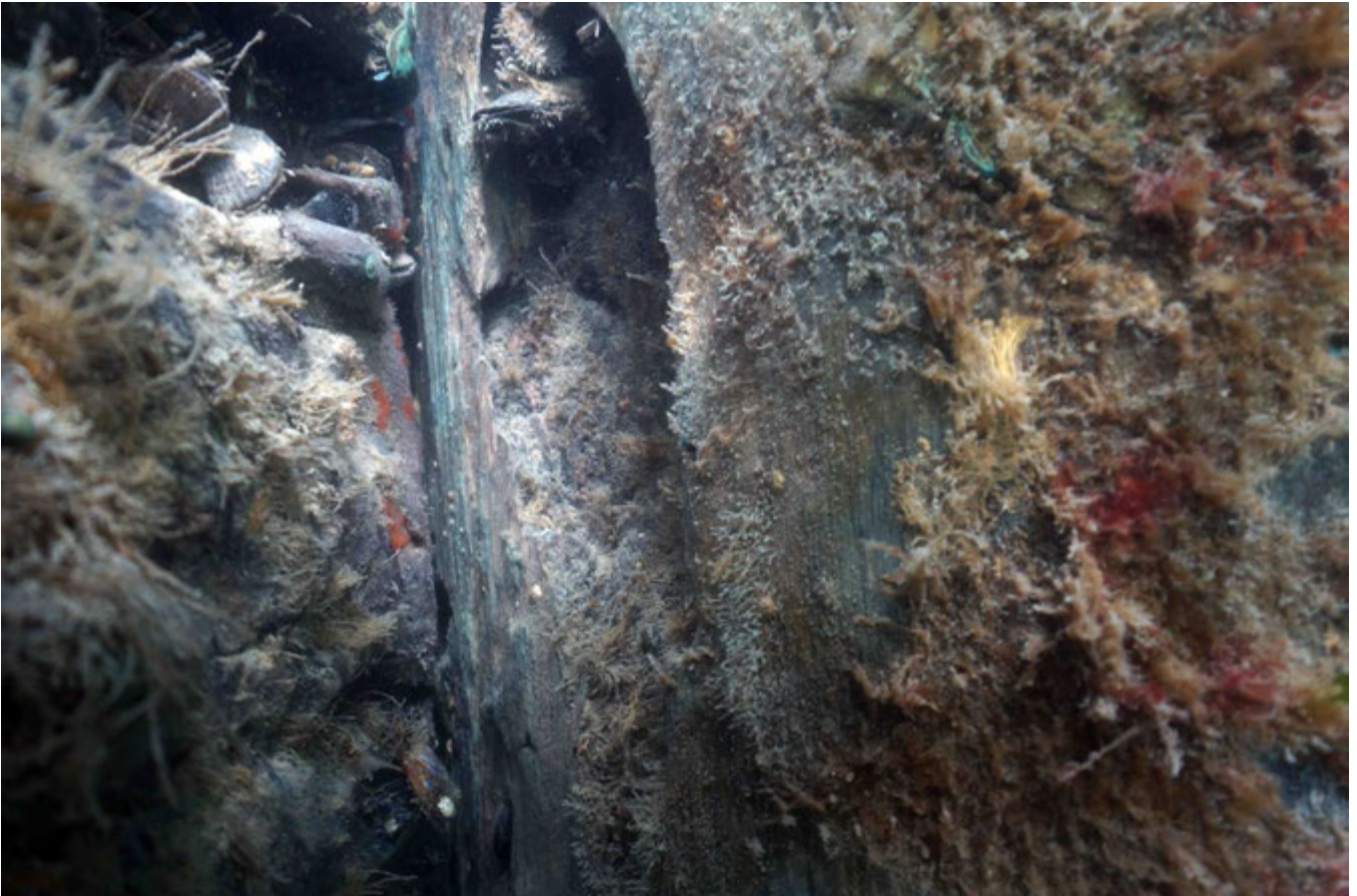
Pile 38D: Poor Condition – 35% loss of section – above tidal zone. Moderate hollowing & decay
