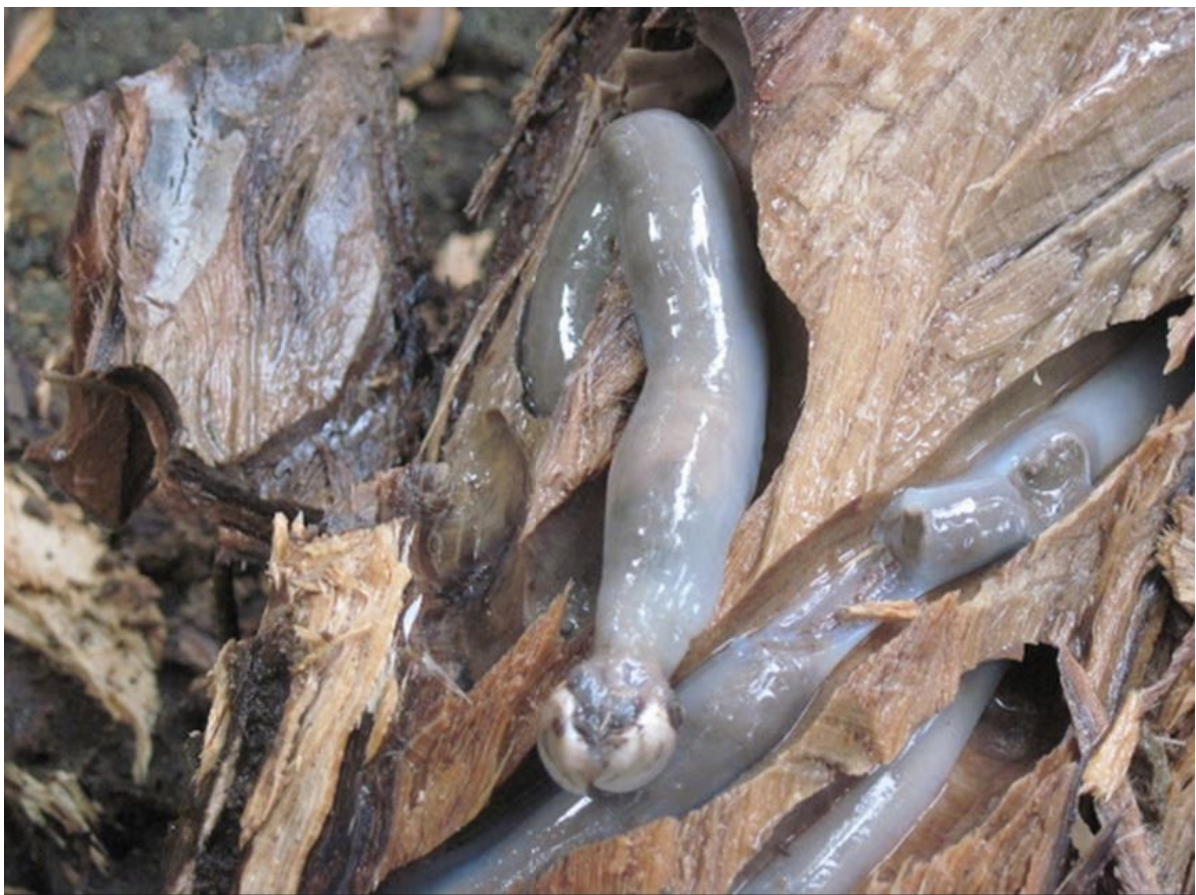
Teredo worm actively destructing a timber pile
