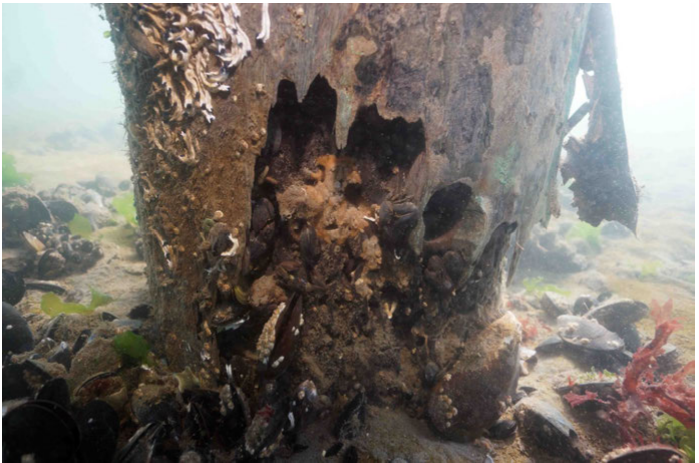
Pile 18D: Poor Condition – 60% loss of section within tidal zone
