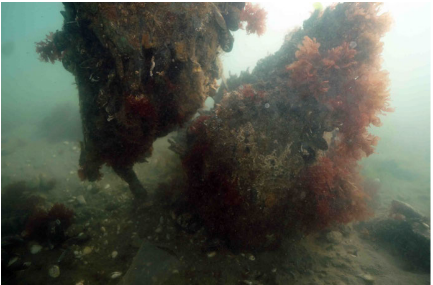
Pile 23C: Very Poor Condition – broken pile
