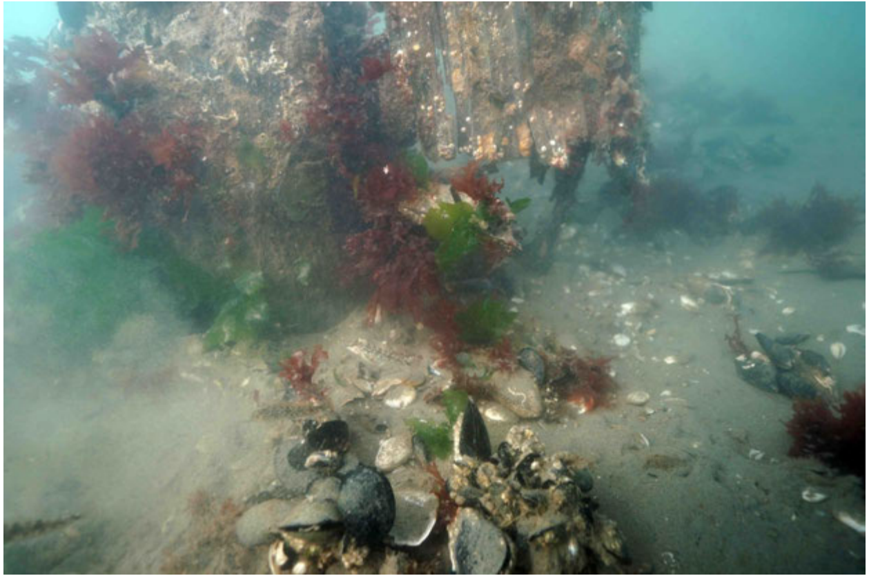
Pile 24D: Poor Condition – 50% loss of section within tidal zone
