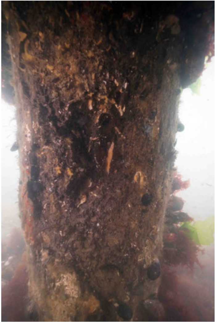
Pile 25C: Poor Condition – 40% loss of section within tidal zone. Severe hallowing
