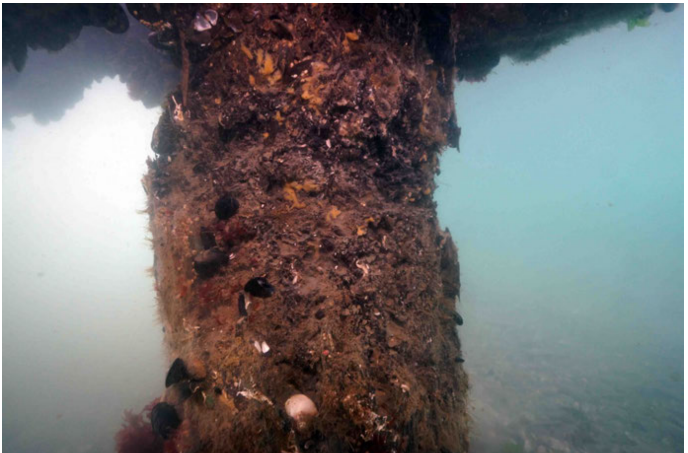
Pile 27D: Very Poor Condition – broken pile
