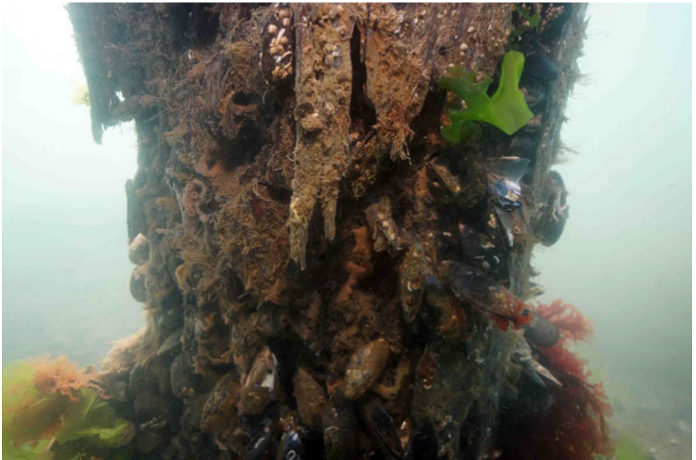
Pile 23C: Very Poor Condition – broken pile
