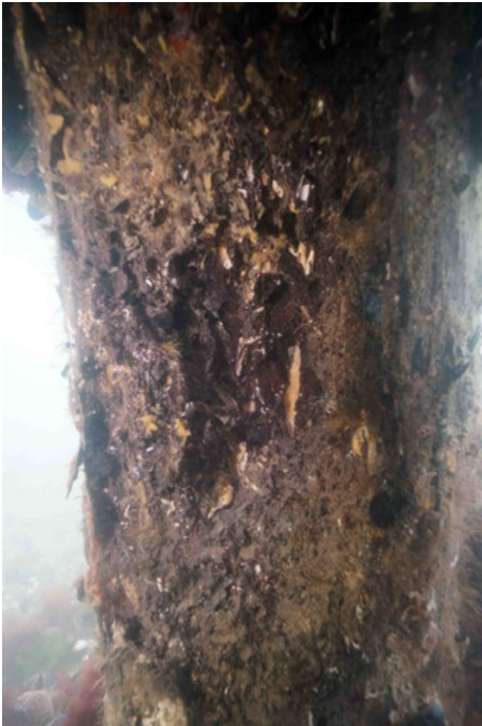
Pile 24D: Poor Condition – 50% loss of section within tidal zone
