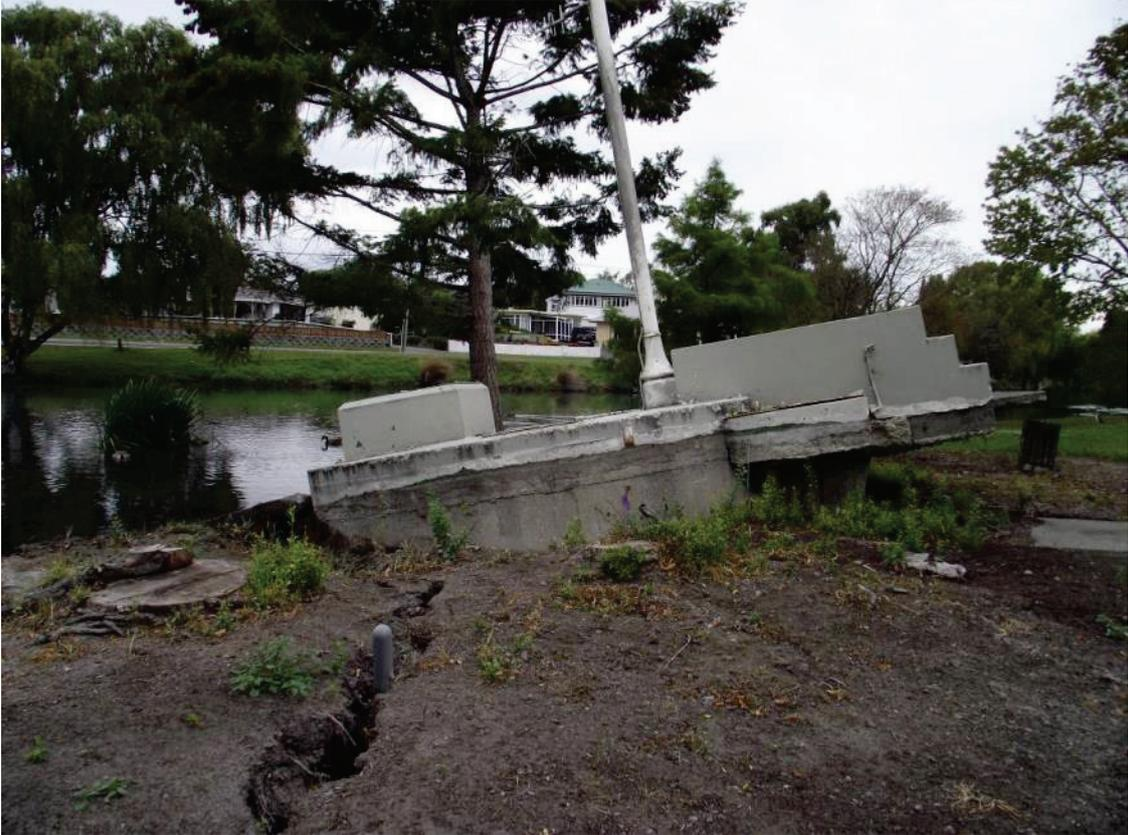
**Photograph 2.3** Buoyancy of a pump-station floated up to 500 mm out of the ground by liquefaction adjacent to the Avon River near the eastern end of Morris Street, approx. 10 km from the epicentre after the magnitude 6.3 Christchurch earthquake of 22 February 2011 (Photo D. Beetham, GNS Science).
