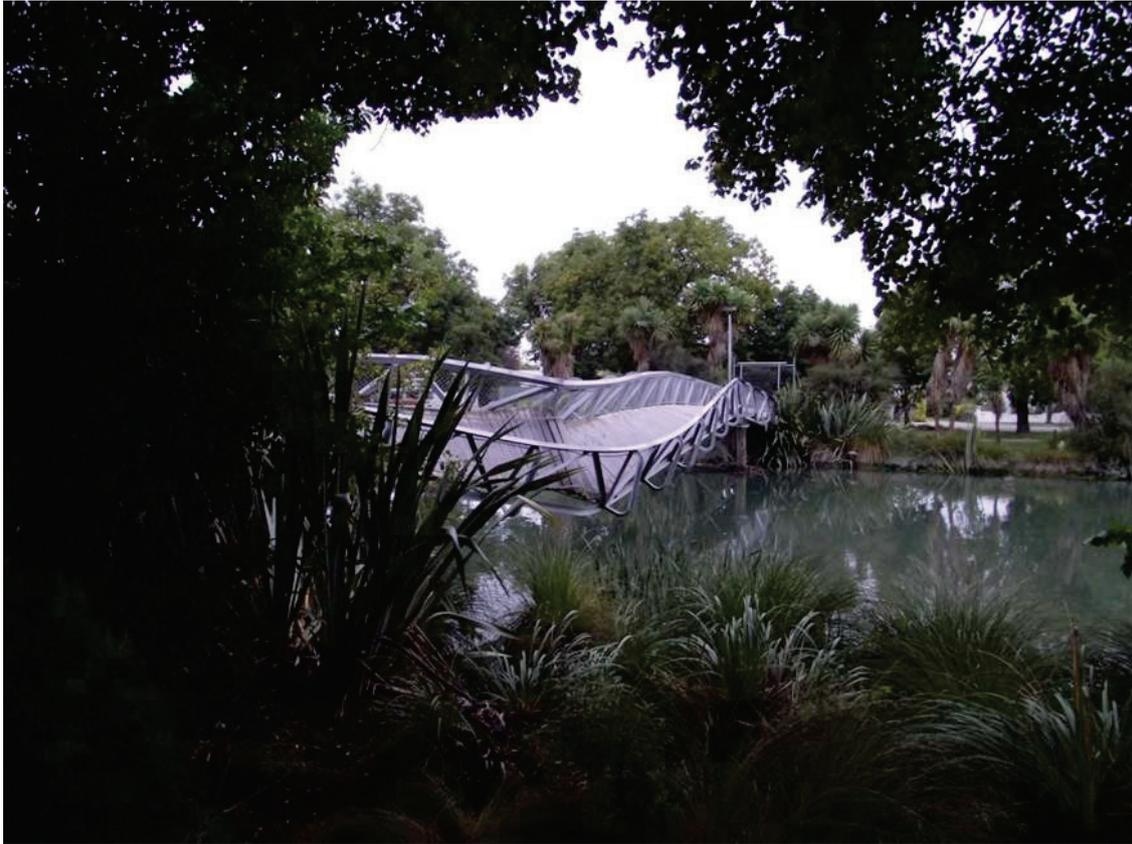
**Photograph 2.5** Compression-induced buckling of a bridge over the Avon River near Medway Street due to lateral spreading displacement of the abutments approx. 10 km from the epicentre after the magnitude 6.3 Christchurch earthquake of 22 February 2011 (Photo D. Beetham, GNS Science).
