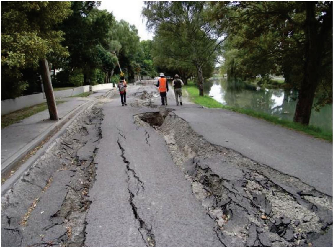
**Photograph 2.4** Lateral spreading fissures run parallel to the Avon River in Avonside Drive, Christchurch, approx. 10 km from the epicentre after the magnitude 6.3 Christchurch earthquake of 22 February 2011 (Photo D. Beetham, GNS Science).
