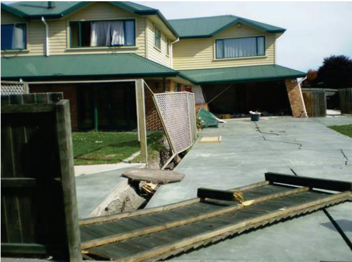
**Photograph 2.6** Liquefaction-induced lateral spreading through the foundation of a house after the magnitude 6.3 Christchurch earthquake of 22 February 2011, location unknown.
