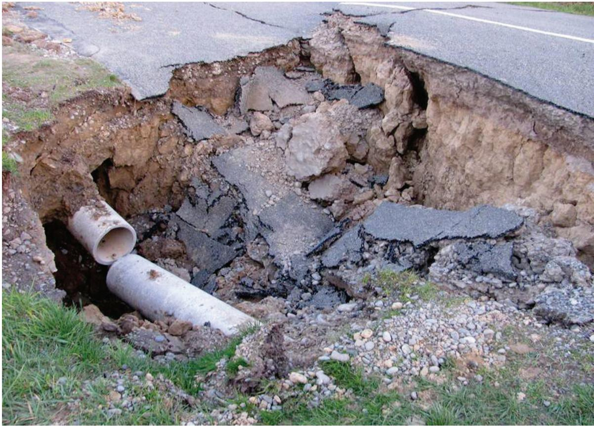
**Photograph 2.7** Damage to underground infrastructure from liquefaction, in this case lateral spreading has pulled a pipe joint apart in Avonside Drive after the magnitude 6.3 Christchurch earthquake of 22 February 2011.
